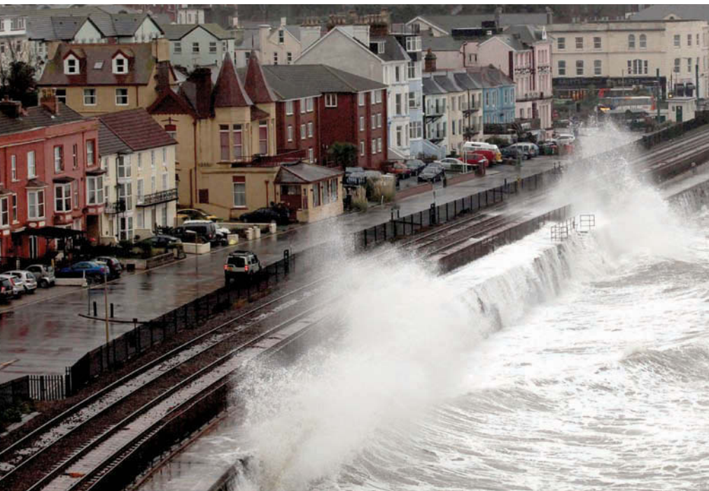
◀ Figure 10.43 Overtopping of the seawall at Dawlish, Devon
