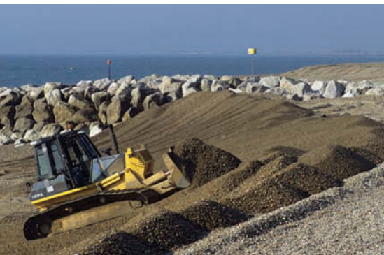
▲ Figure 10.46 Reprofiling
