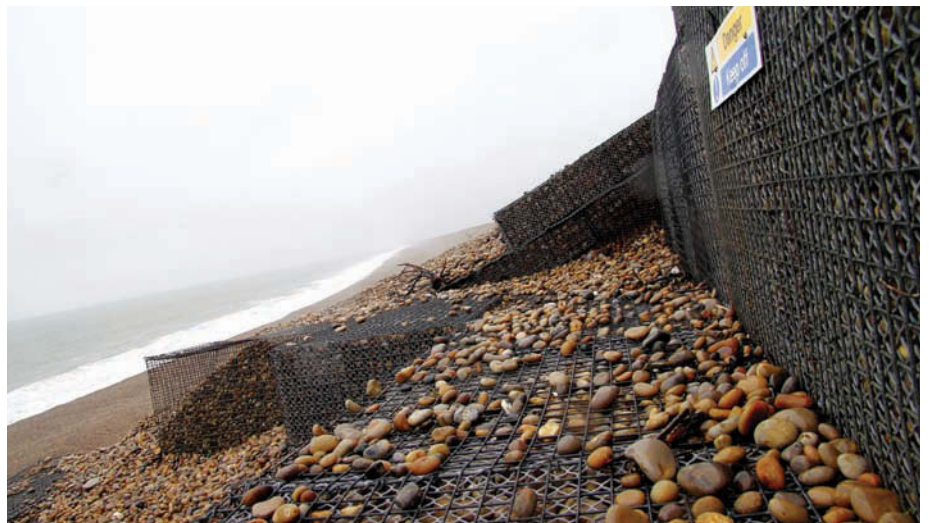
▶ Figure 10.44 Collapsed gabions are unsightly and dangerous
