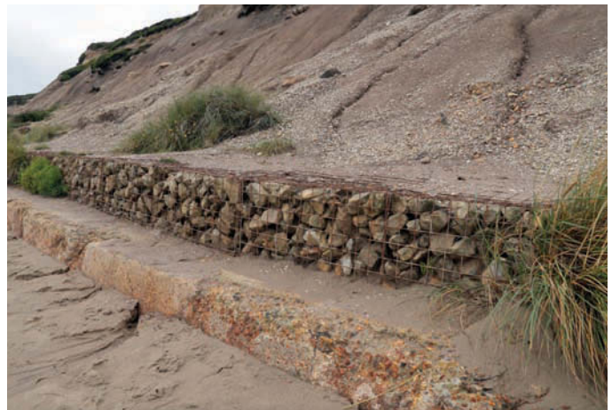
▲ Figure 10.41 Gabions near Hengistbury Head, Hampshire
