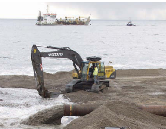
▲ Figure 10.45 Beach recharge at Poole
