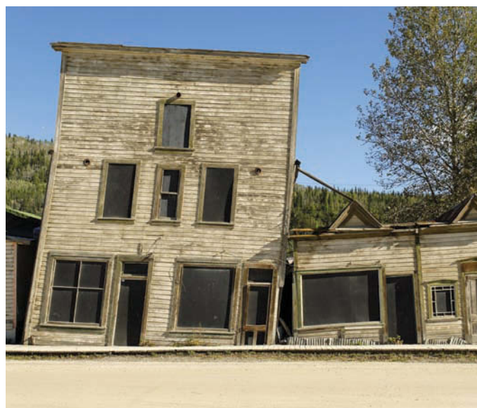
▲ Figure 8.16 House destroyed by permafrost melting, North America
