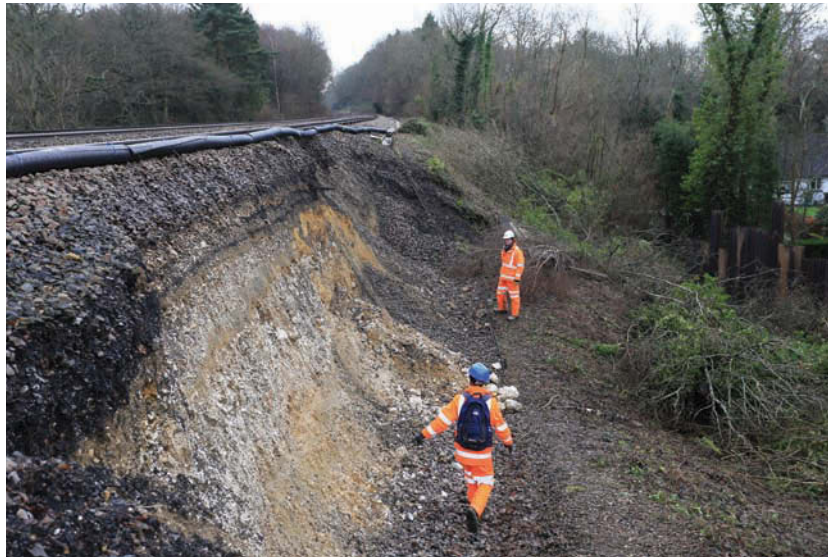
▲ Figure 3.20 The collapse of Ockley embankment after severe storms in 2013
